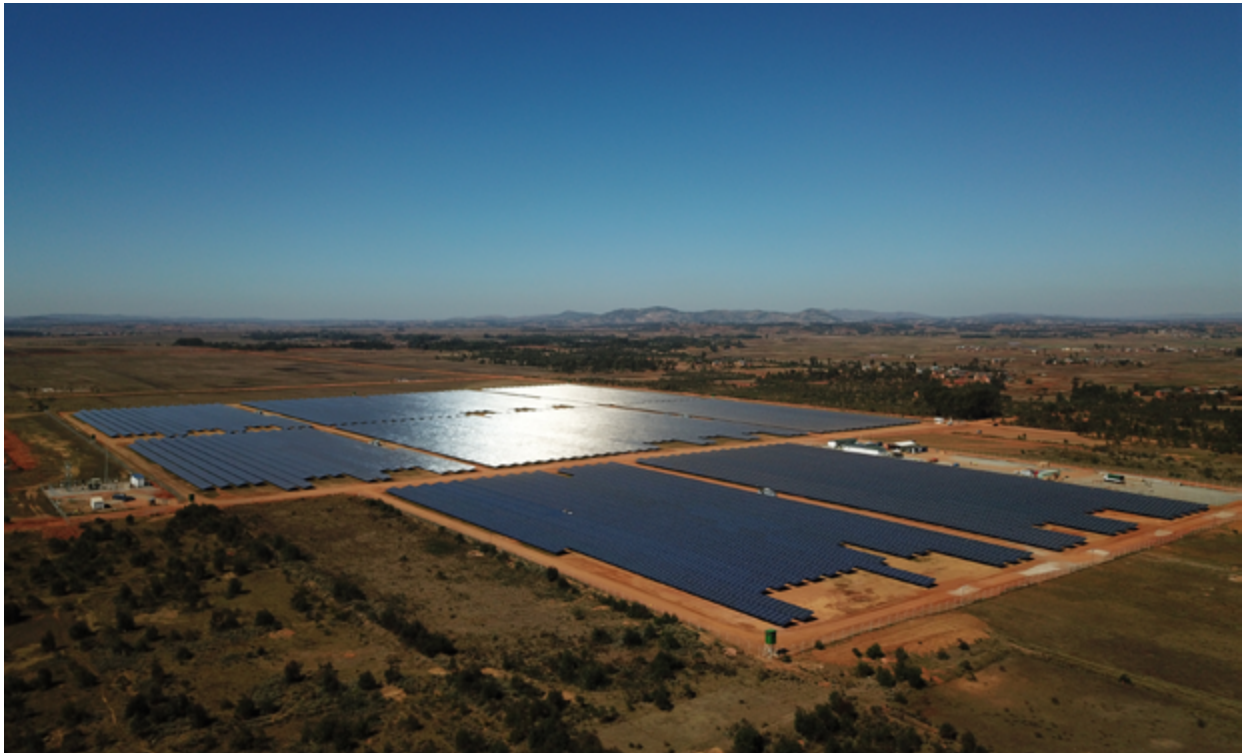
The largest Malagasy ground-mounted solar plant of Ambatolampy built by GreenYellow (20 MWP)
